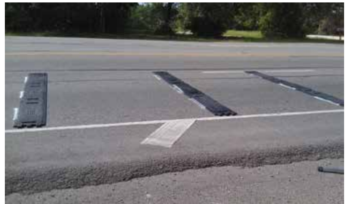
Figure 56. Temporary Rumble Strip Arrays (Source: TxDOT WZ (RS)-16)
