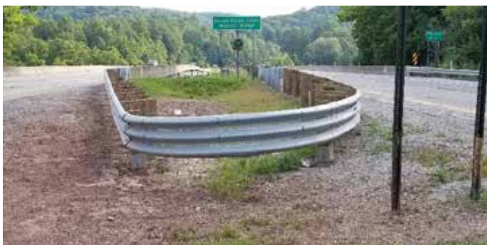
Figure 10. Shielding Bridges with Bullnose median barriers (Courtesy of WVDOT)
