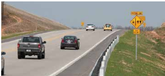
Figure 18. Median Passing Lane CLRS (Courtesy of MoDOT)
