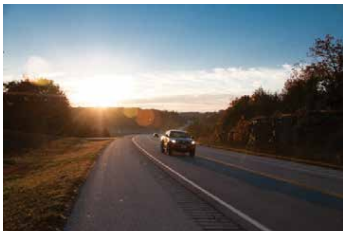
Figure 1. Better guidance with pavement markings and rumble strips (Courtesy of Missouri Department of Transportation)
