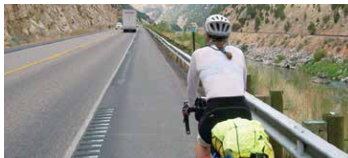
Figure 22. Nevada Modified SRS Design (Courtesy of NDOT)
