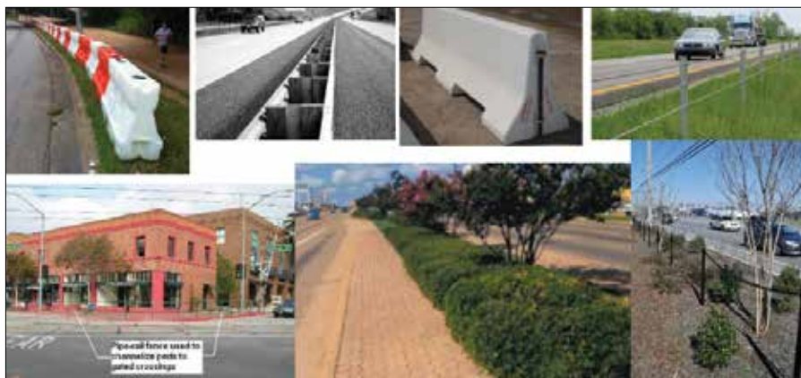
Figure 44. Consideration of Barriers to Redirect Pedestrians (Courtesy of DeIDOT)
