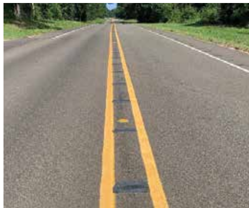
Figure 24. Typical Rumble Bar Installation (Courtesy of Paul J. Carlson, Ph.D., P.E., Chief Technology Officer, Road Infrastructure Investment Holdings, Inc.)
