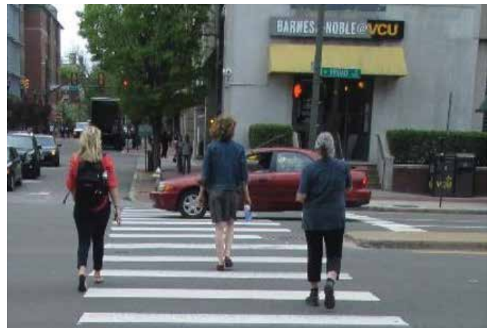
Figure 40. High-Visibility Crosswalks (Courtesy of VDOT)
