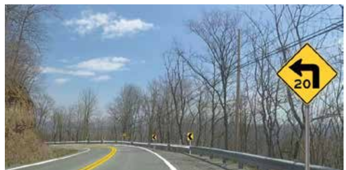
Figure 11. Improved Curve Delineation (Courtesy of WVDOT)
