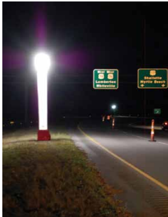
Figure 58. Presence Lighting (Courtesy of NCDOT)
