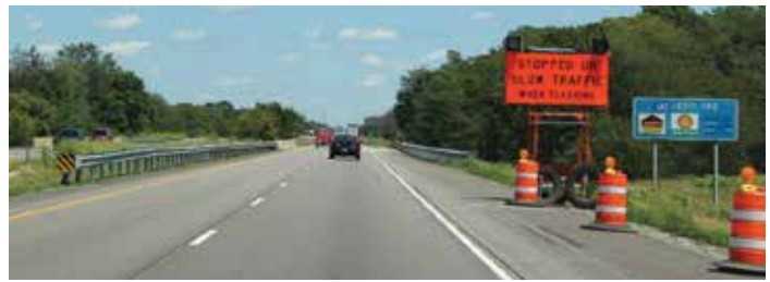
Figure 53. Static Signs with Flashing Lights and Sensors (Courtesy of IDOT)
