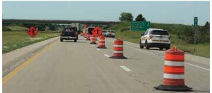
Figure 51. Active Work Zone with Lane Closures (Courtesy of IDOT)
