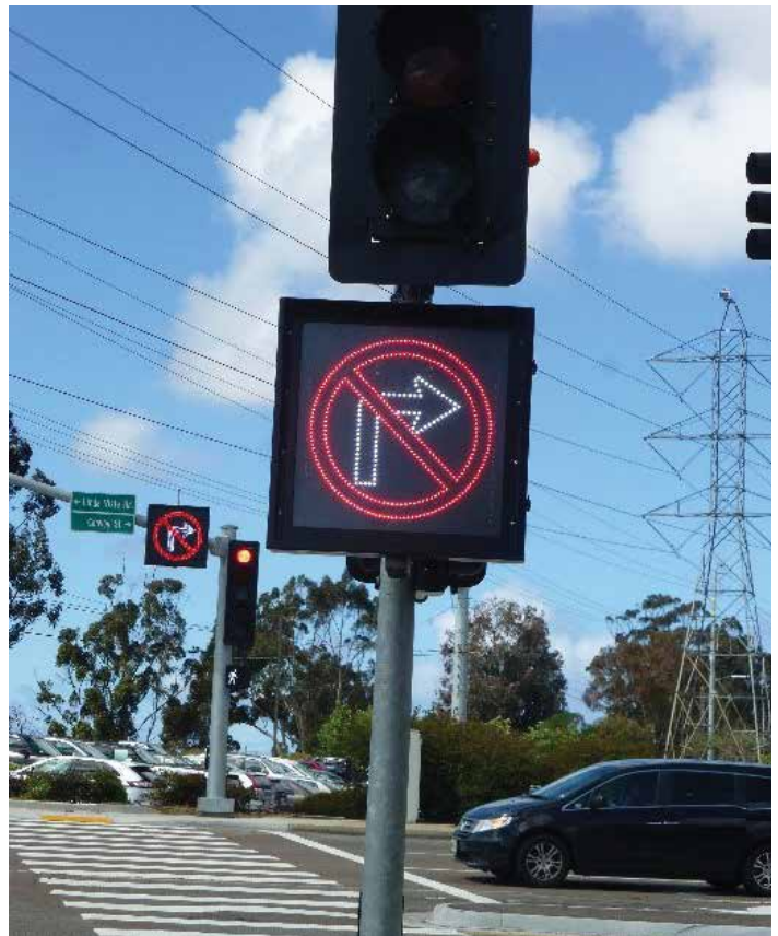
Figure 50. LPI and Electronic Blank-out Turn Restriction Signs (Courtesy of City of San Diego)
