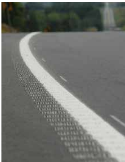
Figure 19. Shoulder Rumble Stripes (Courtesy of MoDOT)
