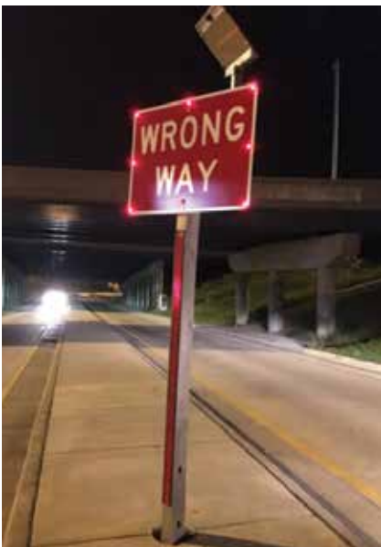
Figure 35. WWD Countermeasure Implementation (Courtesy of WisDOT)
