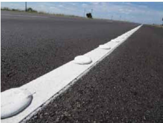
Figure 23. Profiled Pavement Markings 19
